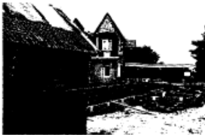
...the rear of Millington Hall
