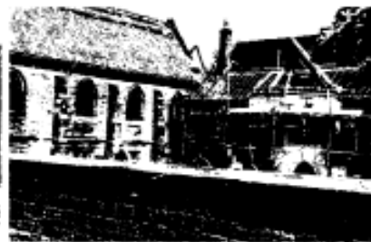
...the rear under construction
